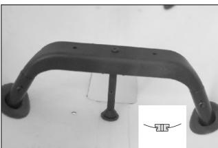
6. Install the lower post which is under the brace, drill 8mm hole and install the Silicon Grommet. Secure the post in place with 3x10mm washer self-tapping screw from bottom and 3x18mm self-tapping screw from top.
