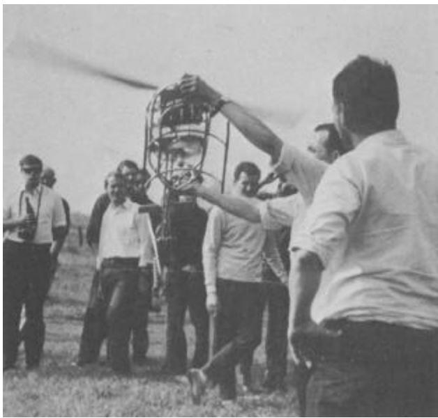
The rotor shaft failed before G. Storig could make an attempt at an official flight with this model featuring aluminum tube construction.
